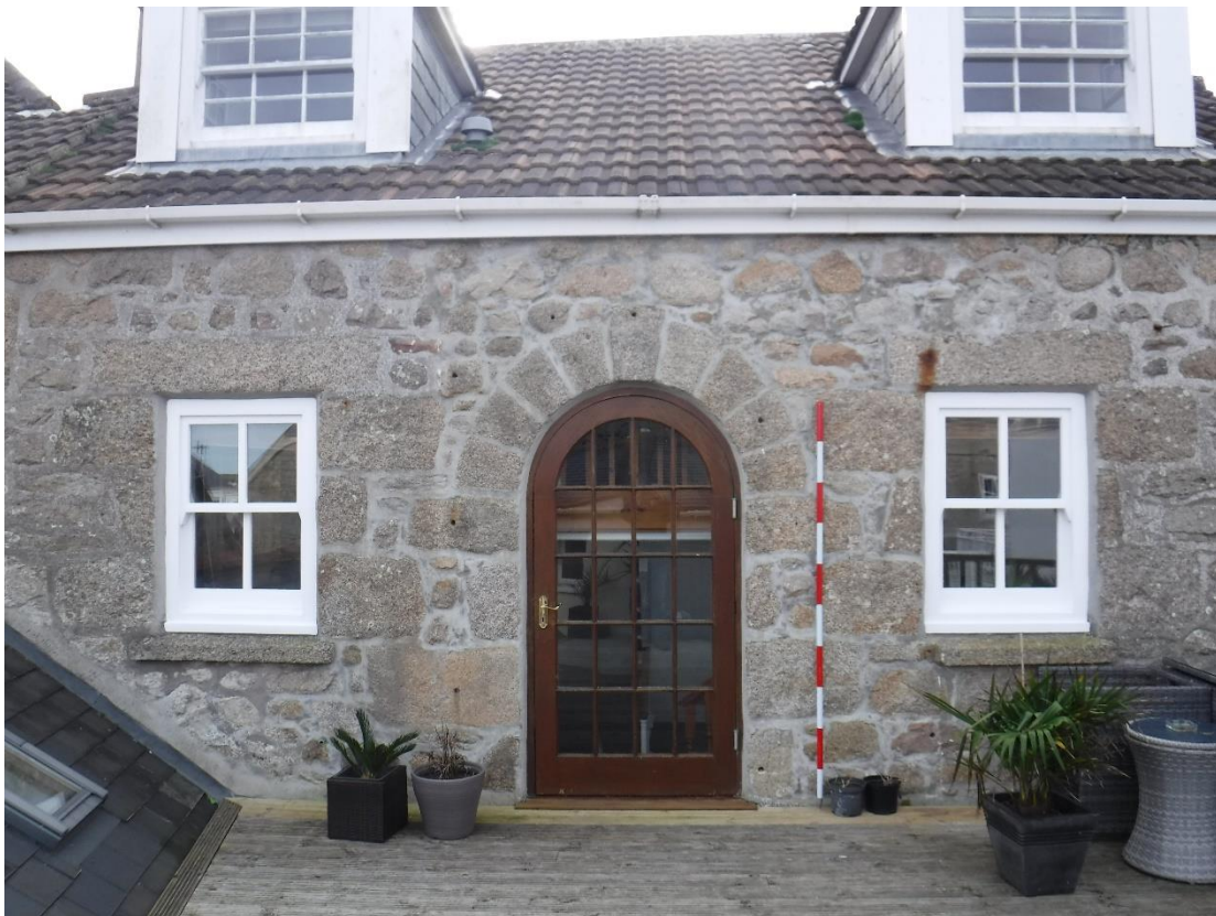
Fig 14 The central window of the first floor rear elevation has been converted into a doorway leading on to a decking surface on the roof of the ground floor extension.
