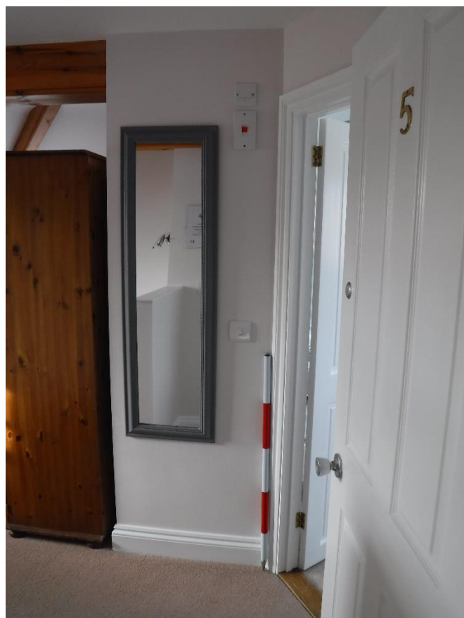
Fig 15 Stud wall concealing chimney breast on first floor.
