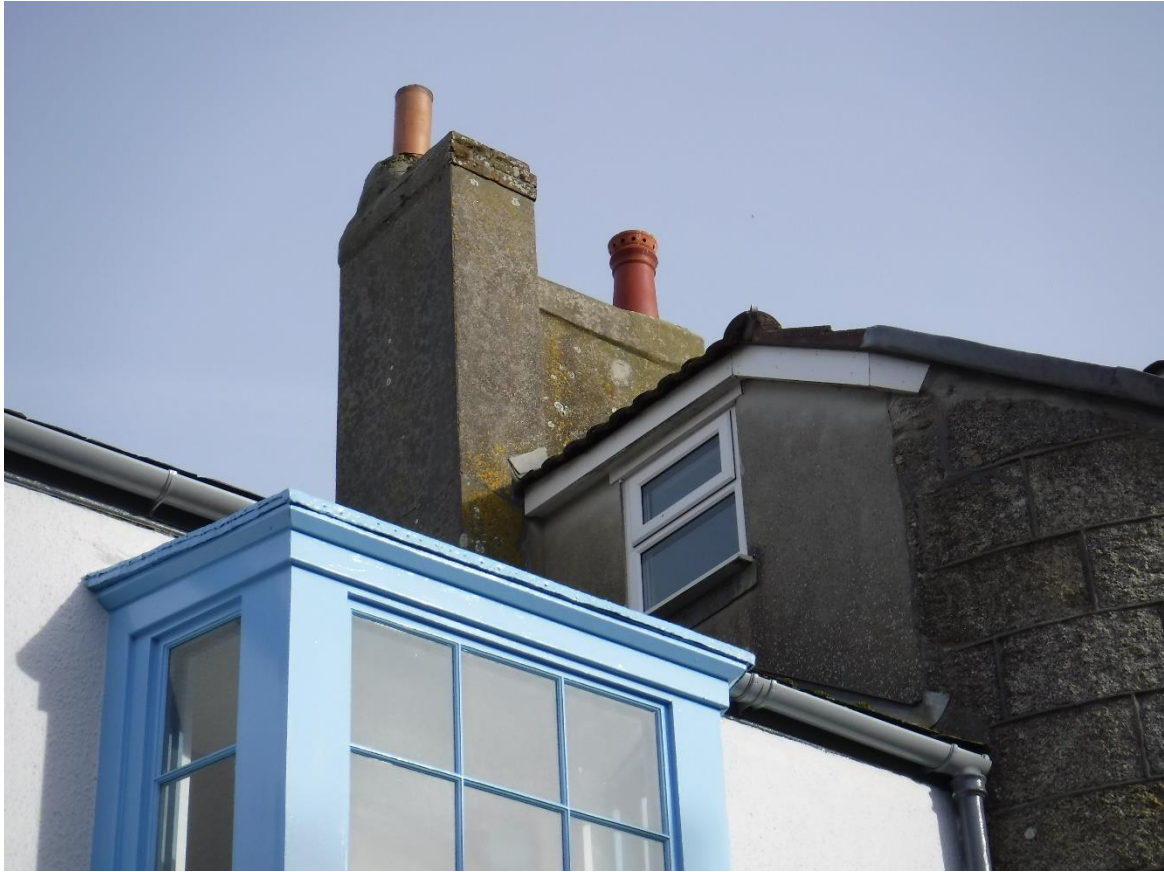
Fig 13 The chimneys at western end of Freesia.
