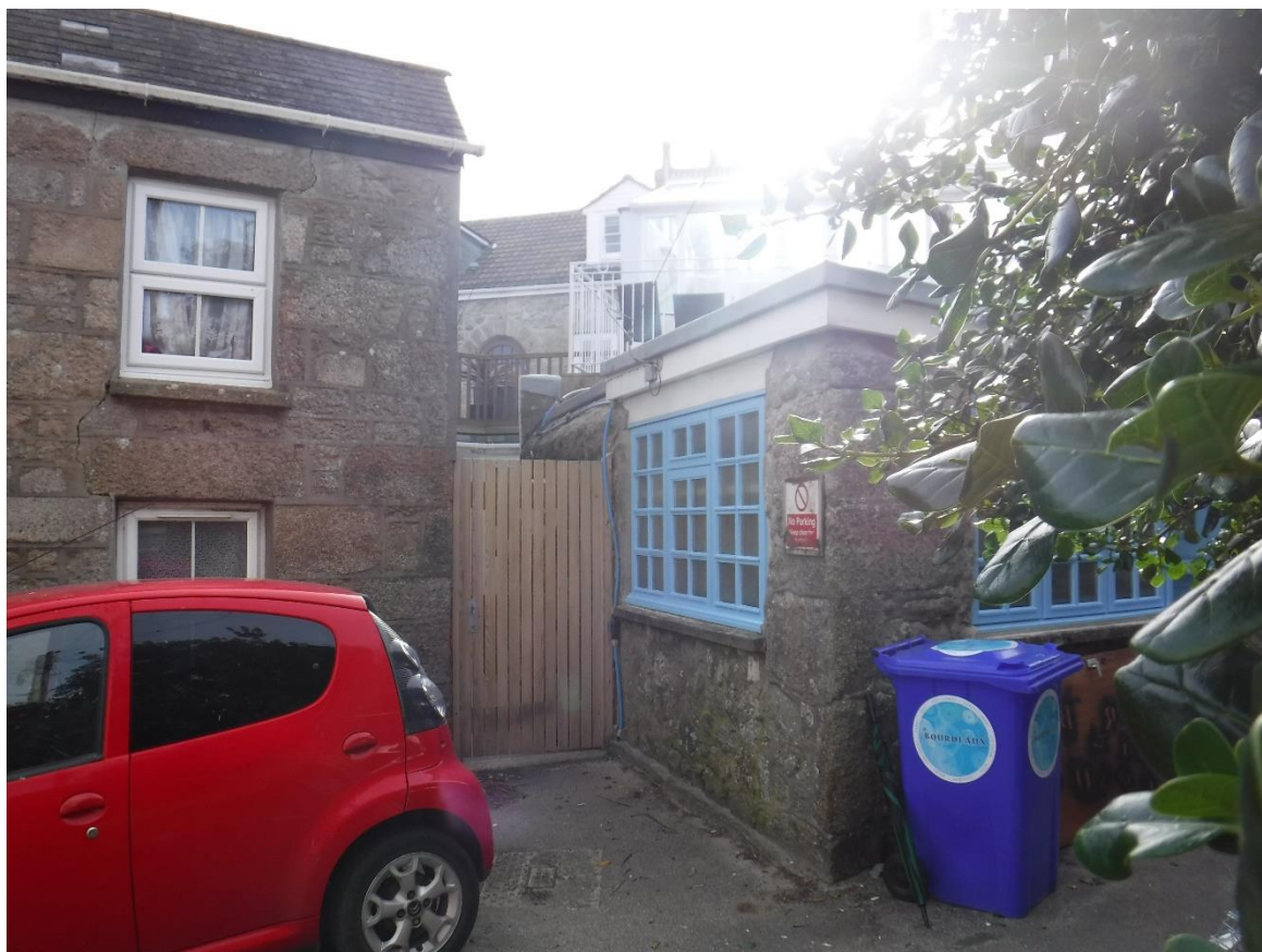
Fig 12 The view of the rear elevation of Freesia from Thoroughfare.
