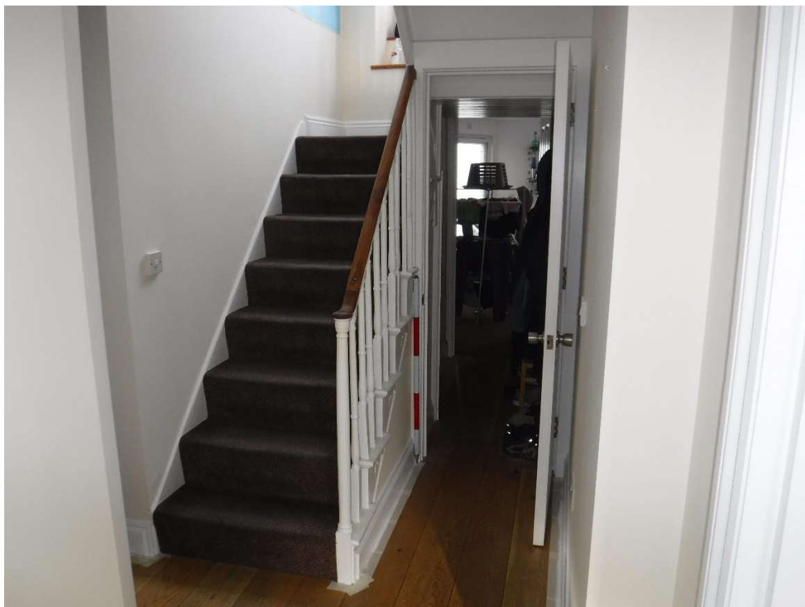
Fig 17 Ground floor staircase.
