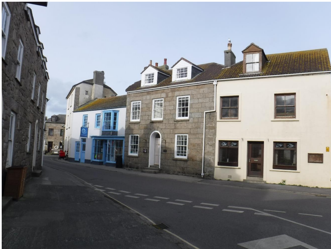
Fig 11 Frontage of Freesia with Bordeaux to the left and Nornour to the right.
