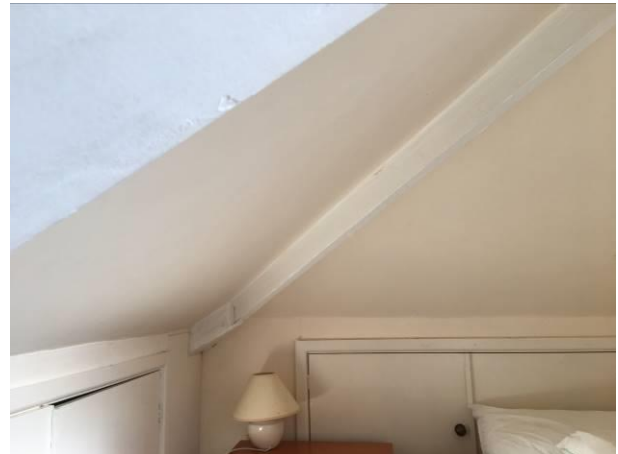
Photograph 4: Showing the interior of the roof space at 1 Buzza Street where the residential conversion has occurred. The built-in storage close to eaves level can also be seen.
