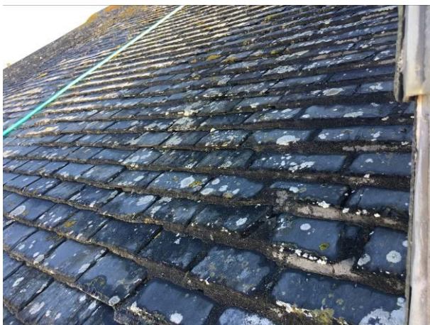
Photograph 5: Showing the tight cement pointing between slate tiles which characterises the roof
