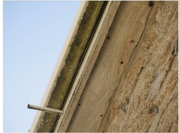
Photograph 2: Showing the underside of the boxed eaves illustrating the tight fitting and lack of access. The guttering attached to a fascia board can be seen to the left.
