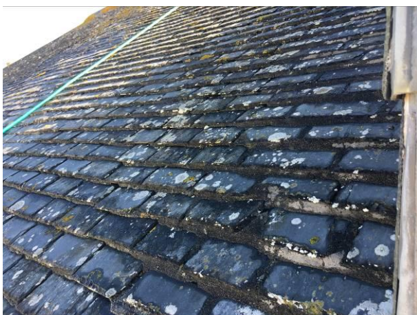
Photograph 5: Showing the tight cement pointing between slate tiles which characterises the roof
