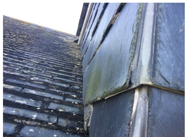
Photograph 6: Showing generally well-fitted hanging tiles of the dormer at 2 Buzza Street – minor cavities have low potential to support individual bats.
