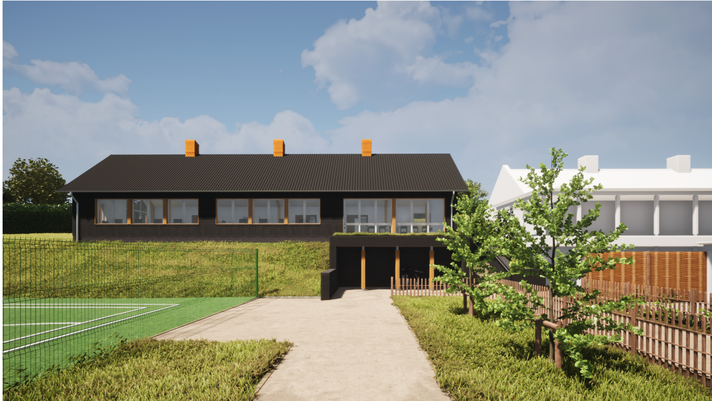
VIEW OF EAST ELEVATION
