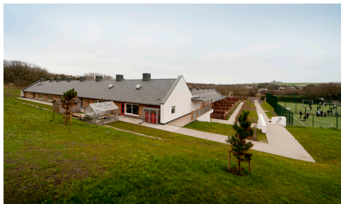
Fig. 05 View A: Existing site context (viewed from west).
