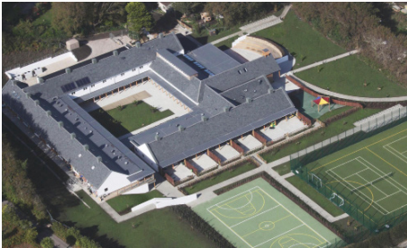
Fig. 01 Aerial view of site.
