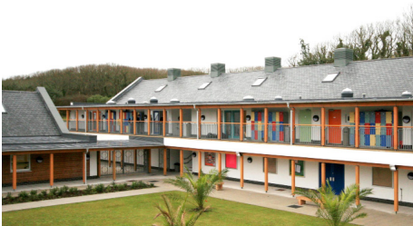
Fig. 02 Existing school building.
