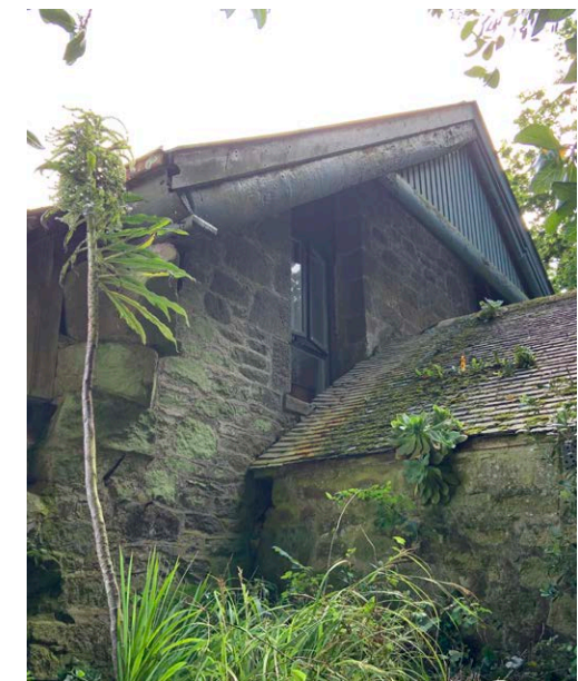
Figure 14. Scantle Roof Detail
