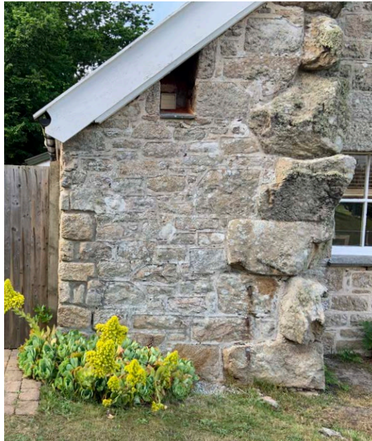
Figure 18. Joint in lean-to masonry
