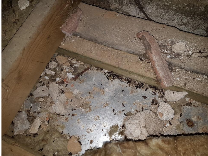
Figure 11: Accumulation of bat droppings at the northern gable end within roof void over the apartment.
