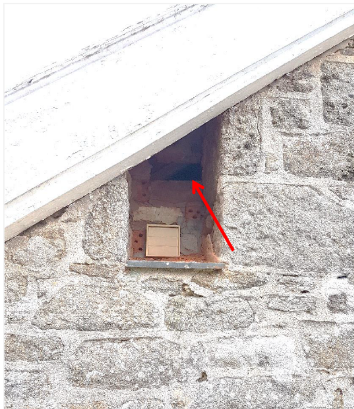
Figure 8: Gap under eaves on southern gable end
