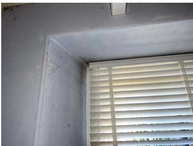
Ground Floor Bathroom Shows damp to reveals and wall at ceiling height
