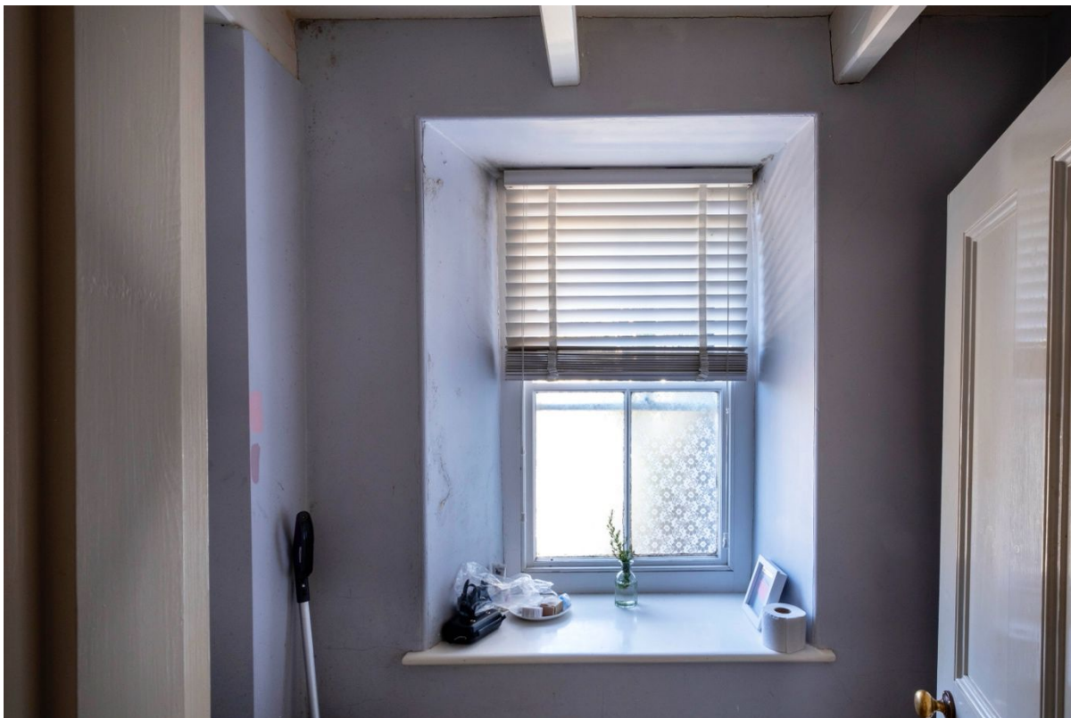
Ground Floor Bathroom Shows damp to reveals and wall at ceiling height
