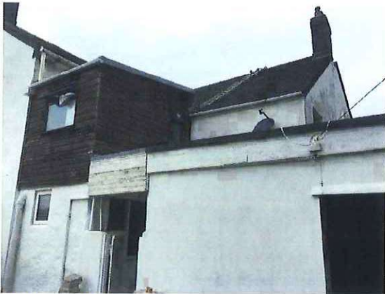
Photograph 9: Showing the garage (bottom right) with the open door visible. The bathroom dormer can be seen to the upper left of the image.
