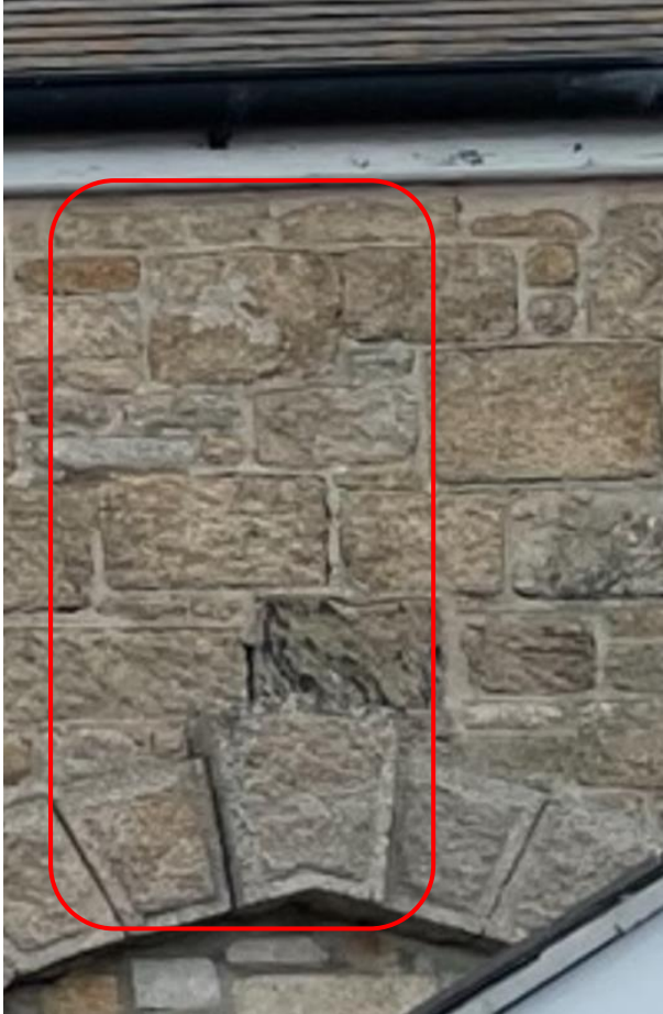
Photo 7 - vertical mortar joints missing
