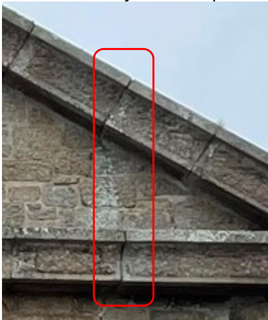
Photo 2 - mortar joint loss in pediment coping projection
