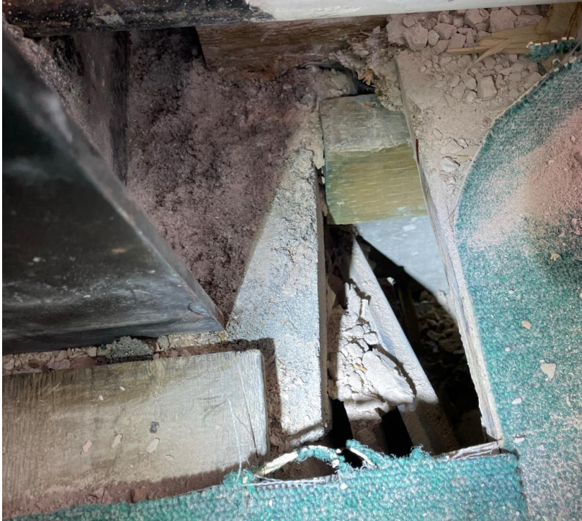
Photo 27 - mansard steel on west side wall cast into top of concrete T beam and T beam cast into ring beam, the face of which is seen under timber joist
