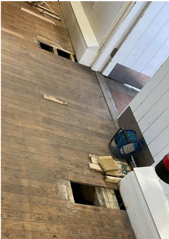
Photo 13 - inspection holes in hall floor
