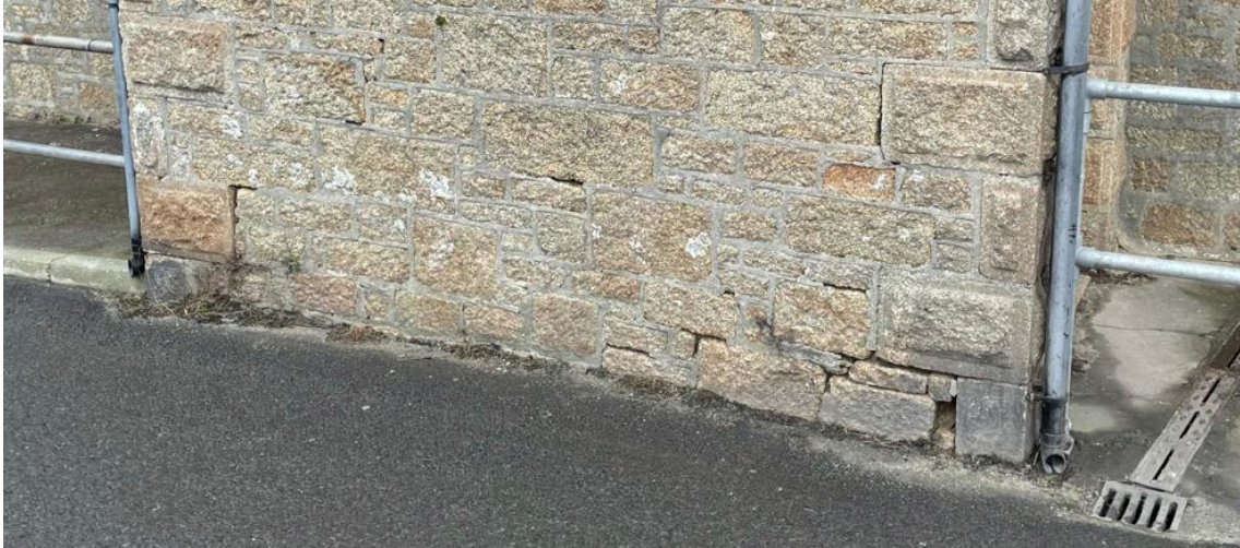
Photo 9 - mortar joint loss on rear porch at ground level
