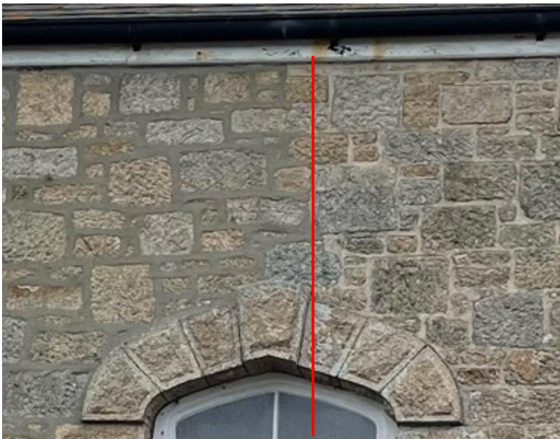
Photo 8 - change of pointing from lime to proud cement in east elevation over south most window head
