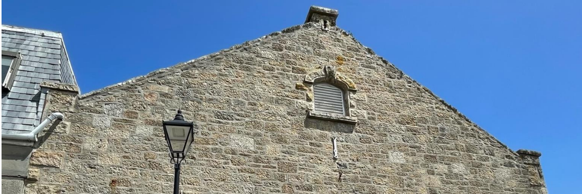
Photo 10 - no coping on south gable. Gutter discharge through gable at eaves
