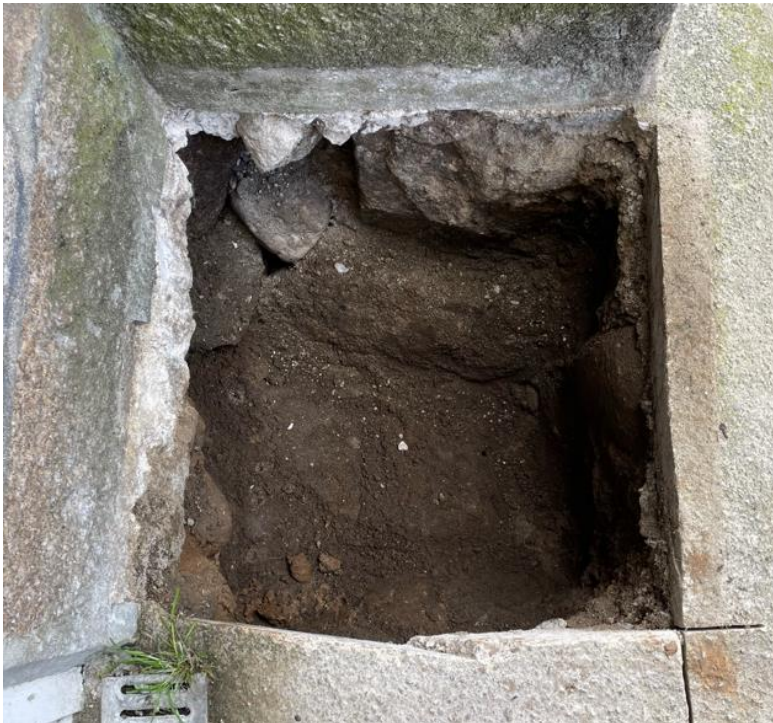
Photo 33 - trial hole at boundary wall with adjacent house to the west on The Parade
