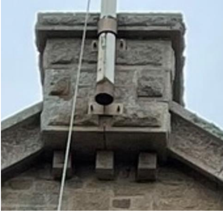
Photo 5 - gable peak pediment block supports cantilever flagpole
