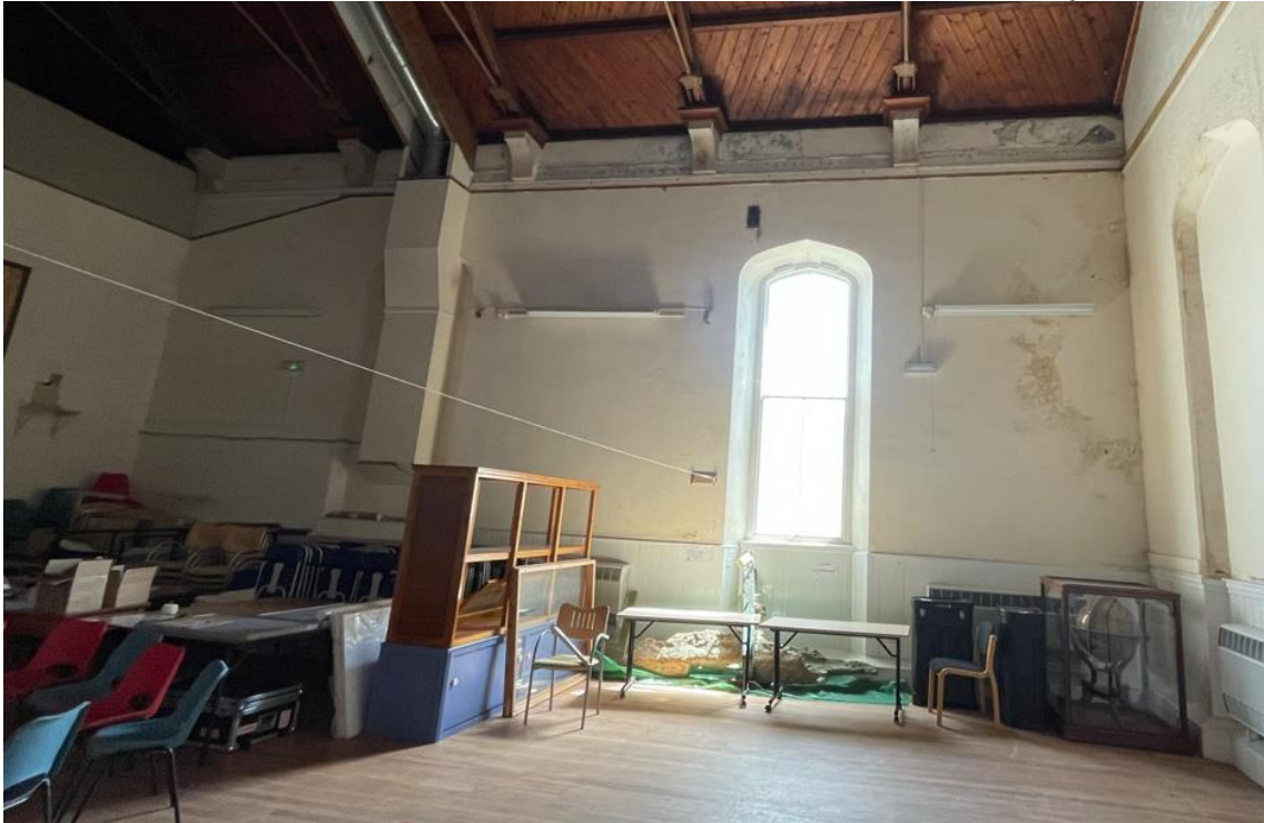
Photo 17 - Main hall west elevation - blocked window at boiler flu position
