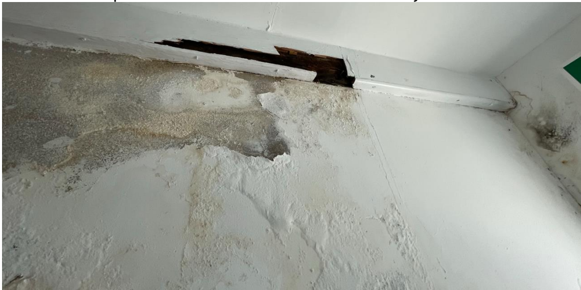
Photo 30 - damp wall at GF rear of office section - decayed timber at FF level
