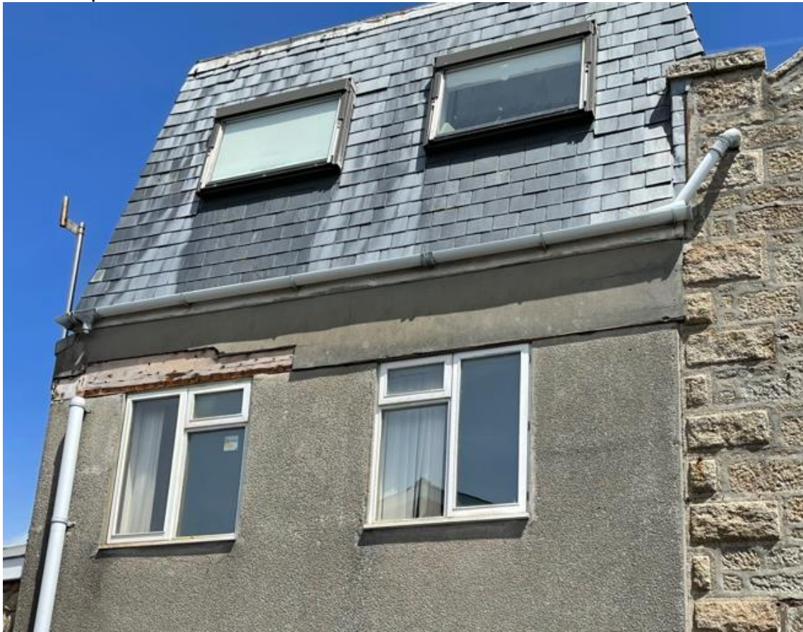
Photo 29 - loss of render over window and pavement below. Joint between render and stone likely allows water to track in creating damp conditions in side see photo 30.
