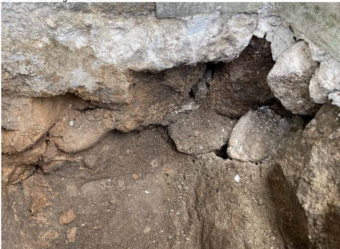
Photo 34 - showing loose stone makeup in foundation. Mortared joints commence at ground level
