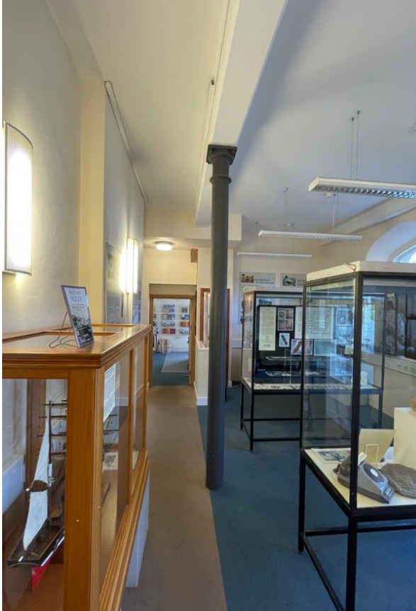
Photo 12 - cast iron columns supporting beam and FF over
