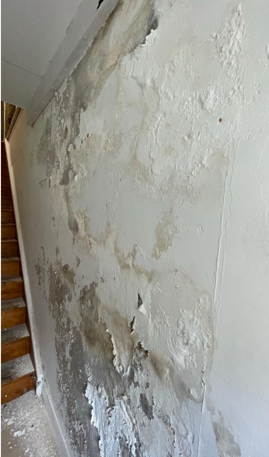
Photo 31 - severe damp in main hall wall - office side GF level
