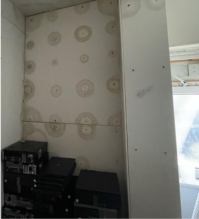
Photo 32 - GF rear storeroom - damp at plasterboard fixings in south elevation
