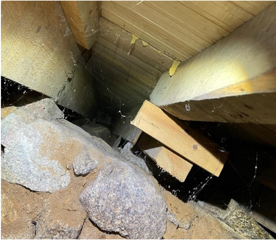
Photo 14 - dwarf walls supporting main hall joists - note poor contact support details
