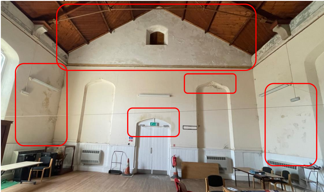
Photo 15 - damp inside south elevation
