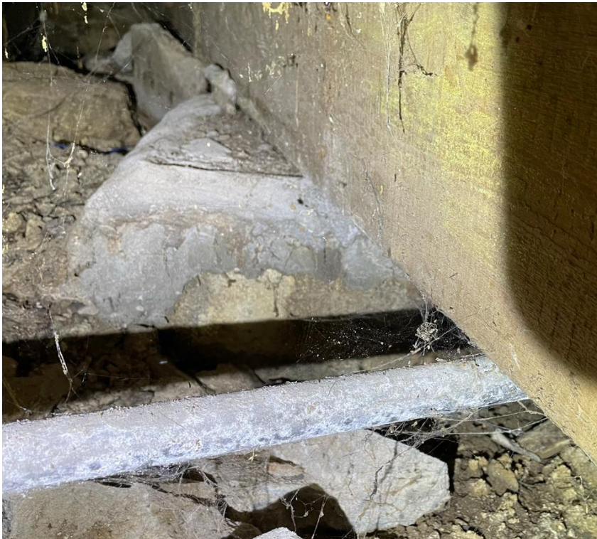
Photo 23 - foul drain access chamber under floor of kitchen
