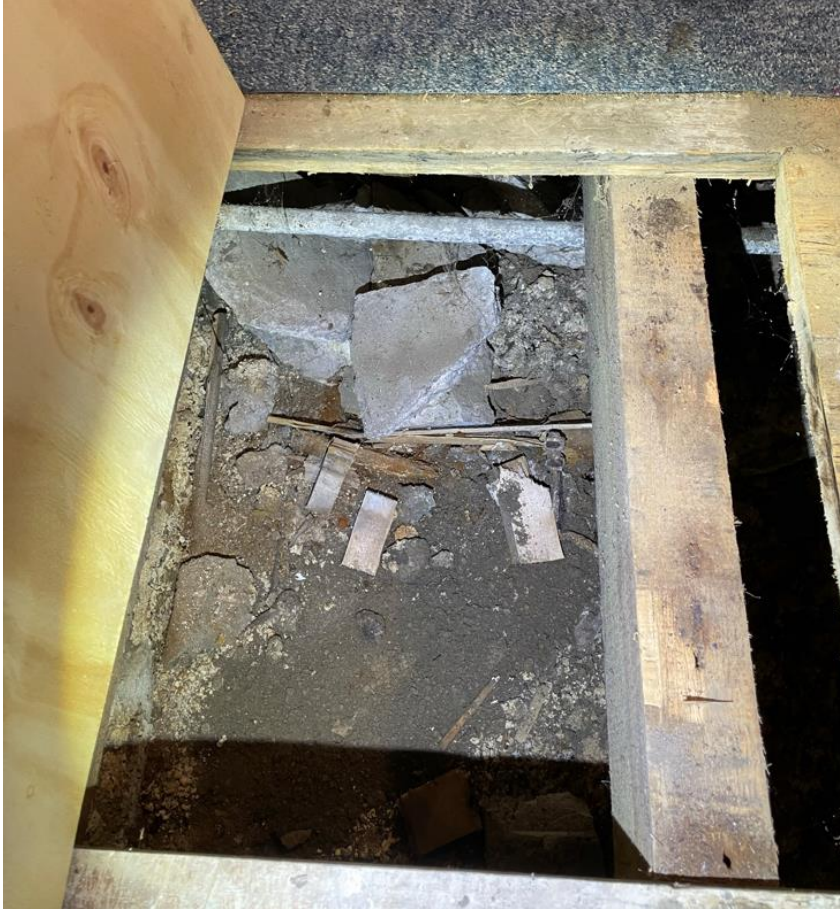
Photo 22 - trial hole in kitchen floor - sand under
