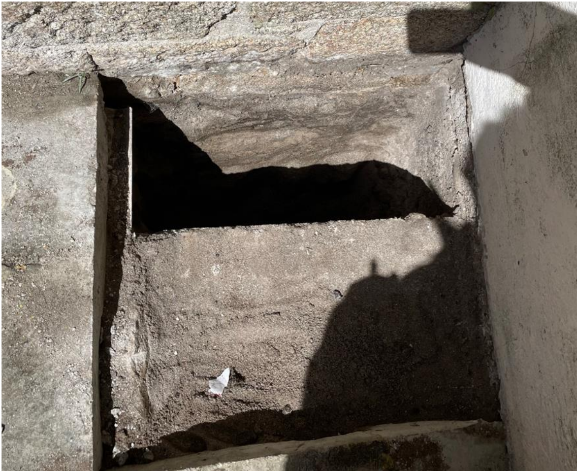
Photo 19 - trial pit west elevation against boiler house and main hall. Note asbestos sheet at left of hole under concrete cap and block wall top of bund and sand in bund
