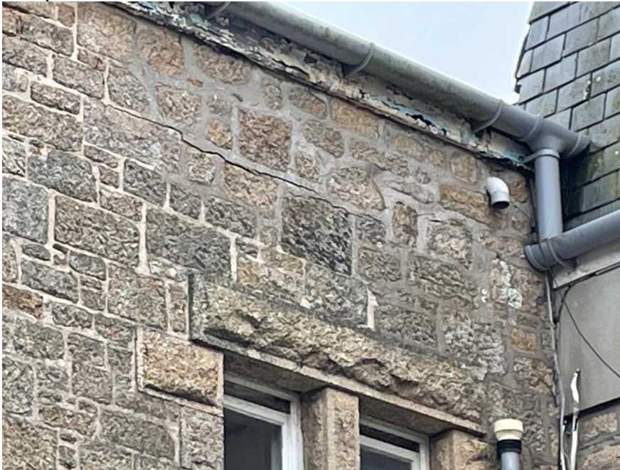
Photo 11 - cracks over high-level window, note repointing and recurrence of crack. Possibly a mirror of the east elevation and buried corroding steel/iron. See photo 6
