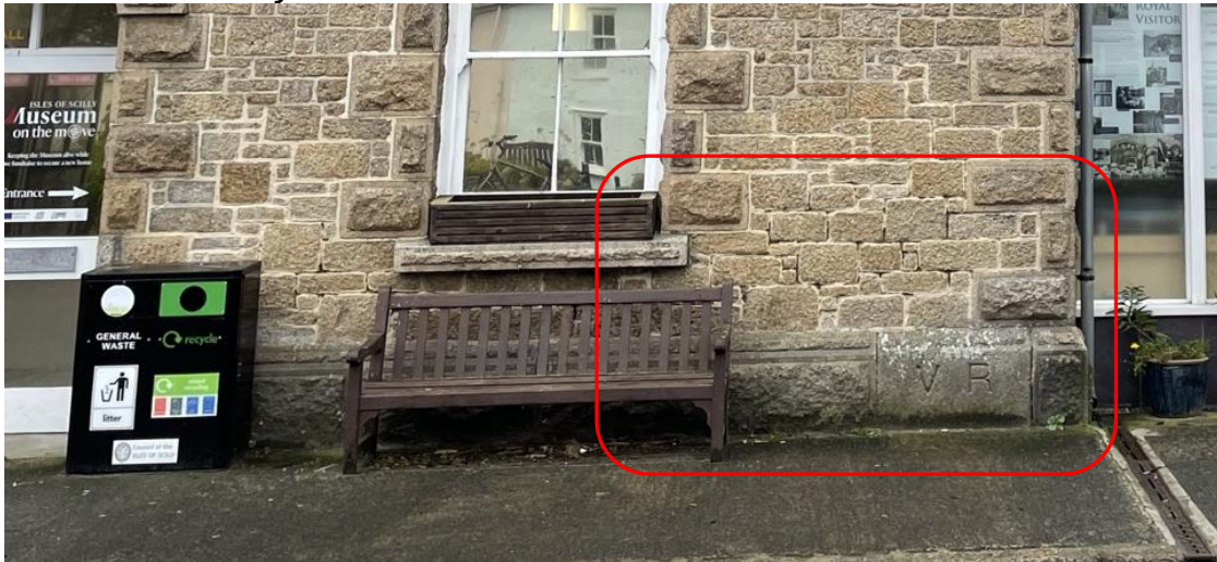
Photo 1 - mortar joint loss
