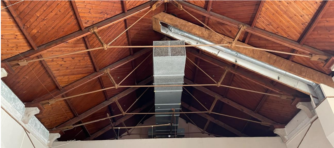
Photo 18 - Exposed roof trusses supporting air duct in main hall.
