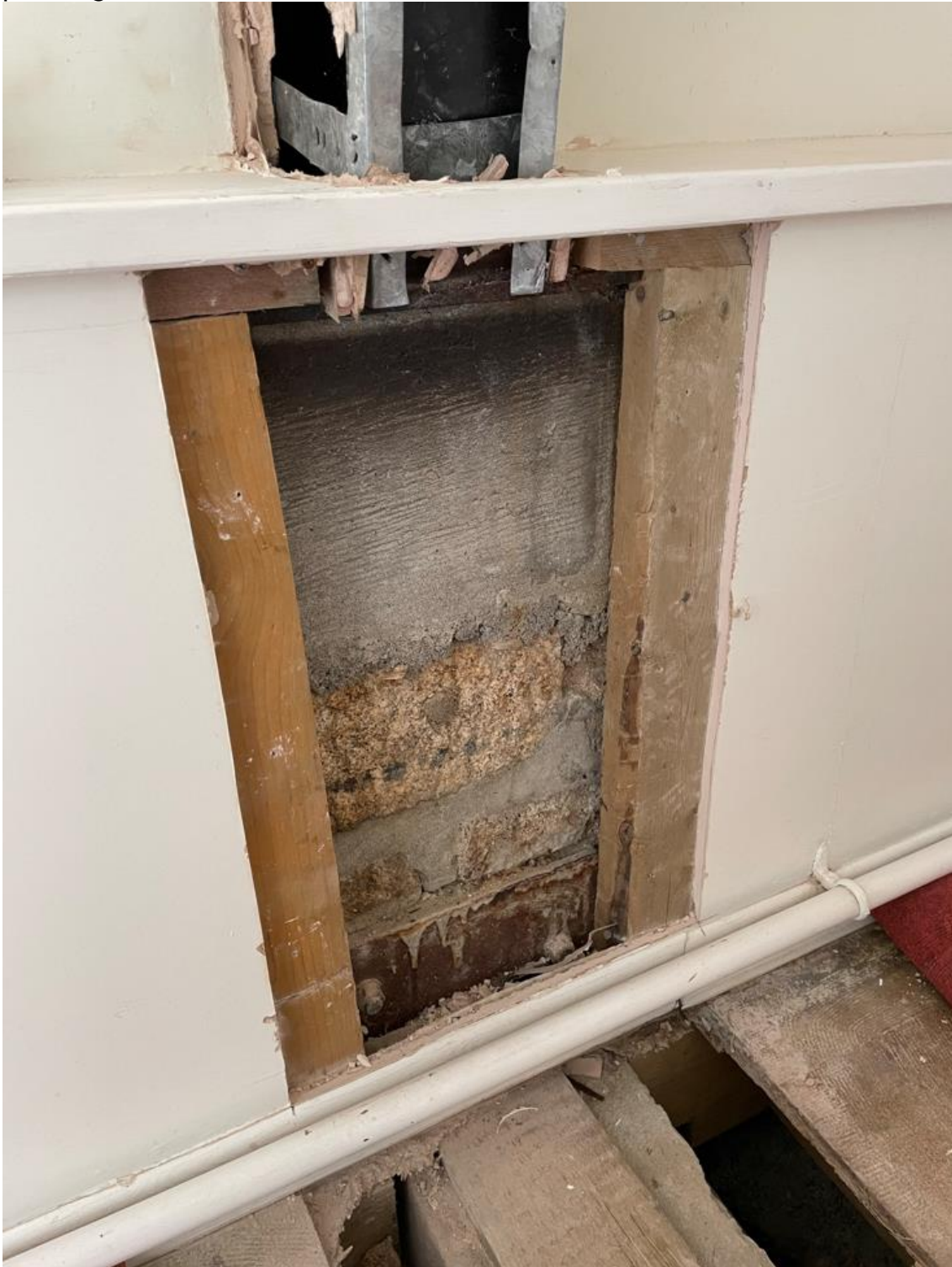
Photo 26 showing mansard steel on main hall wall on concrete ring beam or pad on granite and concrete T beam in the floor zone
