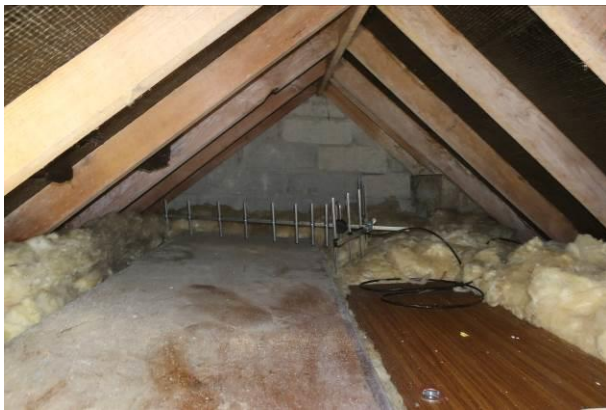
Photograph 3: Showing the interior of the roof space with typical timber rafters and an exposed internal ridge board.
