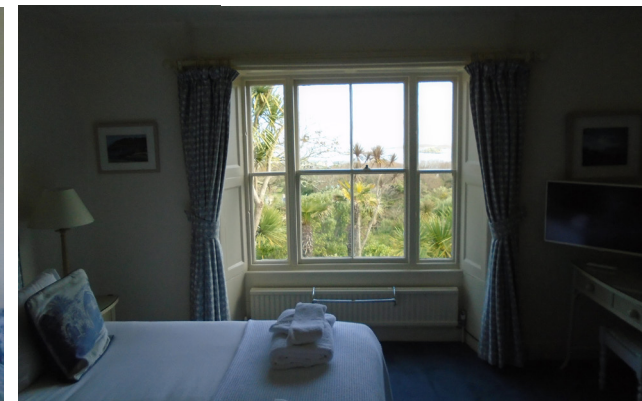
Figure 15 - Original window joinery in bedroom 2 (Tresco Estate)
