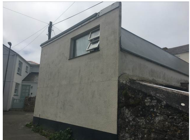
Photograph 4: Showing the eastern façade of the 2-storey extension with the steep single-pitch element which terminates the otherwise flat roof on the northern aspect.
