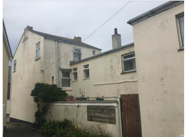
Photograph 2: Showing the southern aspect of the building complex including the single-storey outbuildings and the 2-storey flat-roof extension behind the main 3-storey house.
