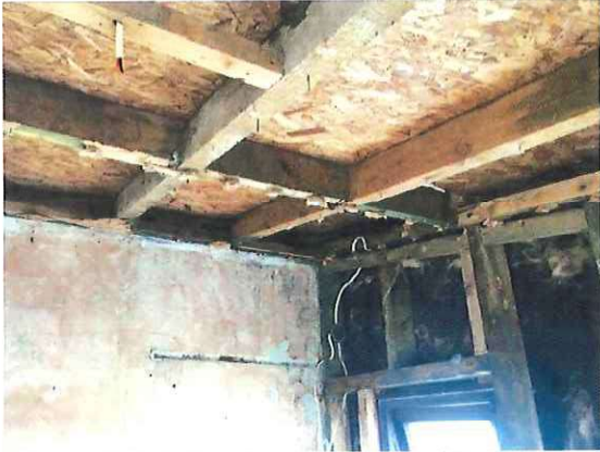
Photograph 1: Showing the interior of the bathroom dormer. The wall of the residential building is visible to the left with the timber frame of the external wall visible to the right. The timber roof structure and chipboard can also be seen above.
