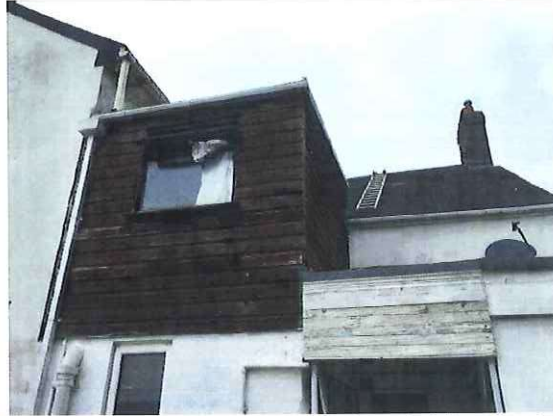
Photograph 2: Showing the timber cladding on the exterior of the bathroom dormer.
