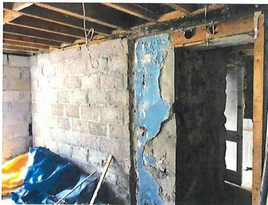
Photograph 10: Showing the interior of the garage with exposed breeze block walls and exposed timber roof structure above.
