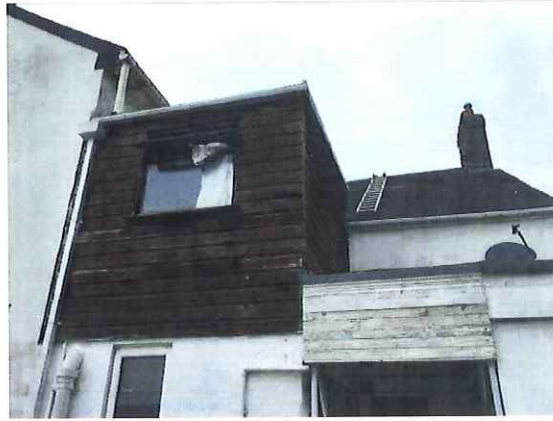
Photograph 2: Showing the timber cladding on the exterior of the bathroom dormer.
