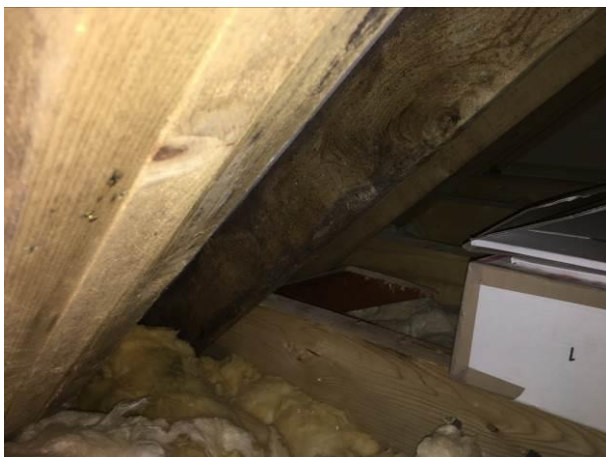
Photograph 5: Showing the interior of the eaves loft space where the new roof of the extension will tie in.
