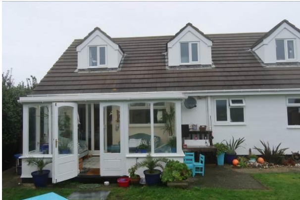
Photograph 1: Showing the property viewed from the south including the conservatory to be demolished.
