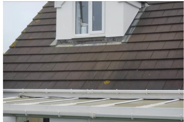
Photograph 4: Showing the pitch of the roof where the new extension roof will tie in – the interlocking concrete tiles are well fitted and in excellent condition.
