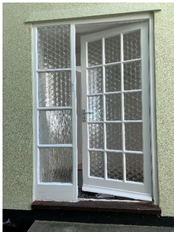
5. Back door and side panel
