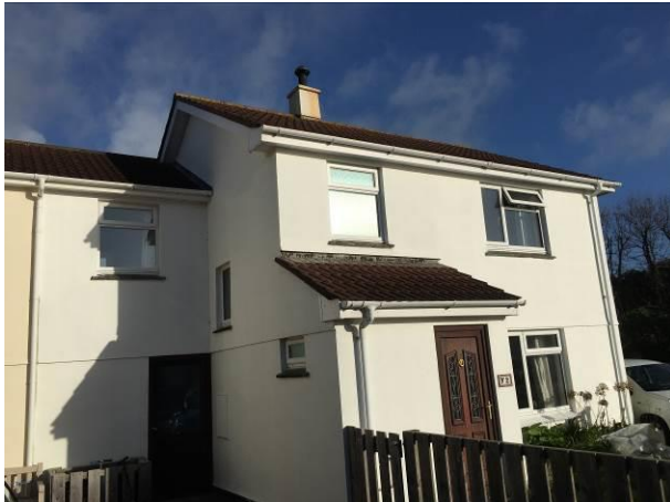
Photograph 1: Showing the property from the front including the porch to be demolished.
