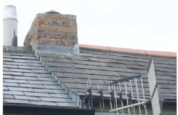
Photograph 2: Showing a closer view of the chimney taken from the east.
