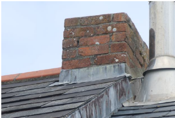
Photograph 3: Showing a closer view of the chimney taken from the west.
