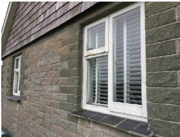
Photograph 3: Showing the wooden windows fitted within the reconstituted stone block walls
