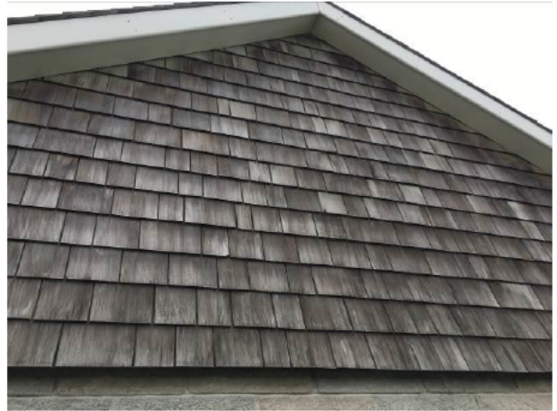
Photograph 2: Showing the shingles on the gable ends of the property
