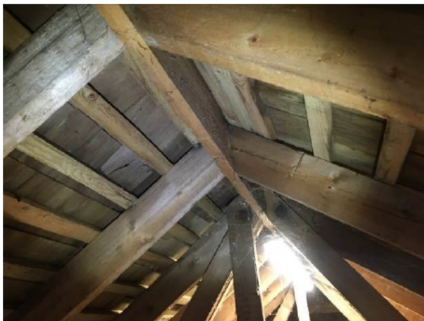
Photograph 5: Showing the roof structure with ridge board visible. The shingles are attached directly to the battens.
