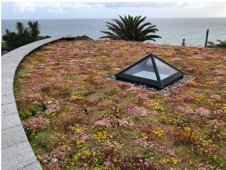
Mixed Sedum roof – Porthmeor View, St.Ives
