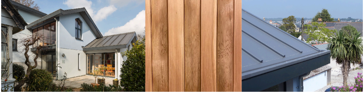
Left: Sarnafil roof cladding with planted battens, Bellair, School Lane, Truro
