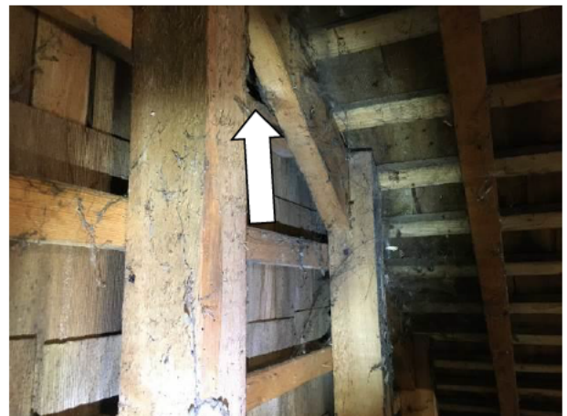
Photograph 6: Showing the apex of the interior gable – an example of the locations where minor gaps are present are indicated.
