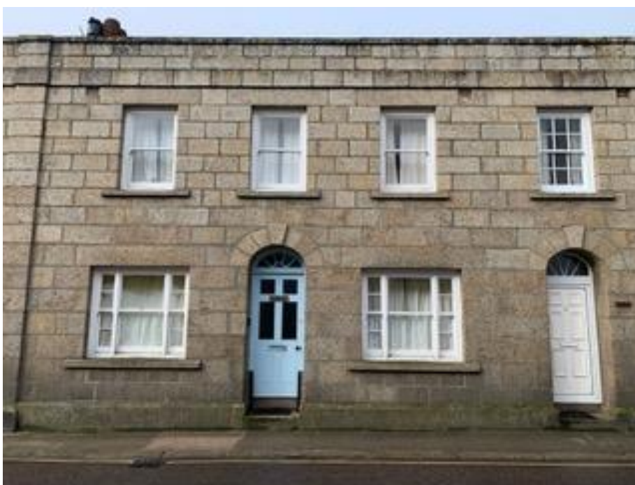
Fig. 1: The north-east, front elevation of St Eia, No. 5 Hugh Street.
