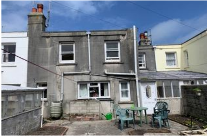
Fig. 6: View, looking north-east, of the existing rear elevation of St Eia.
