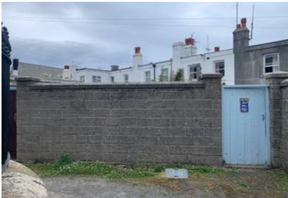
Fig. 23: View, looking north-west, of the rear elevations of adjoining houses of the terrace.
