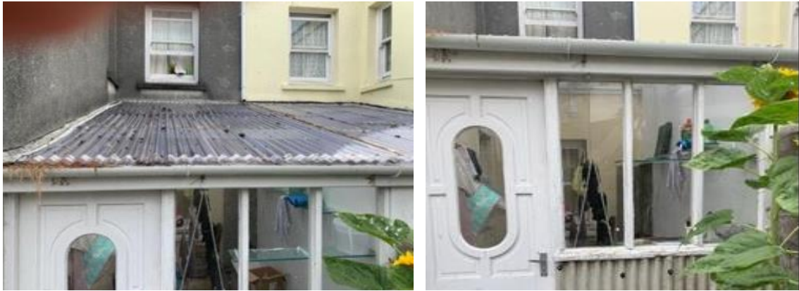
Fig. 18 A and B: The existing rear porch.
