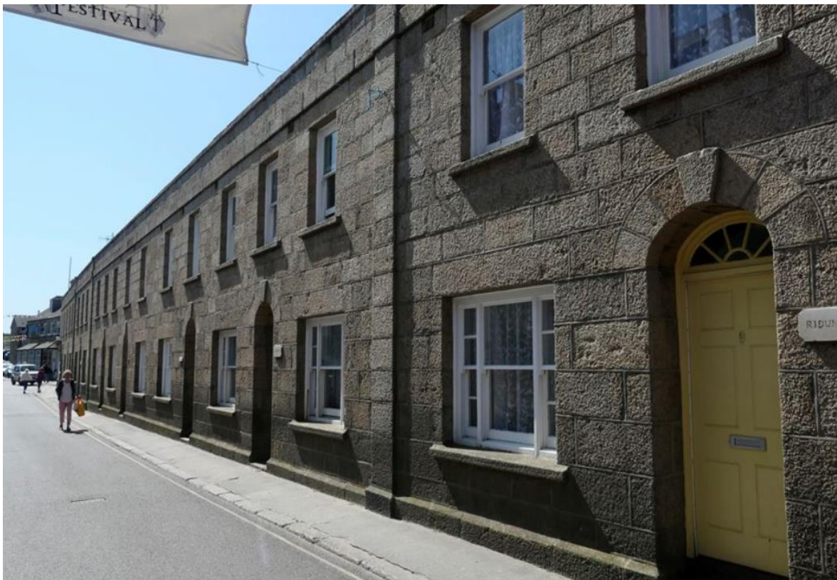
Fig. 5: View, looking south-east, of Nos. 1-8 Hugh Street, with front elevations (Historic England).
