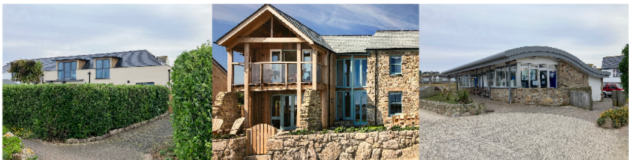
Top: 9 Little Porth. The original roof aligned with number 8 next door Below: Examples of successful contemporary designs on Scilly
