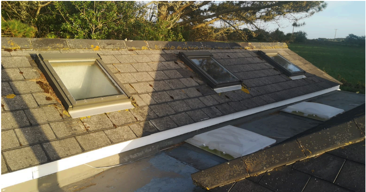
Above: The pitched roof over the garage, corner of the main hipped roof and flat roof connecting link
