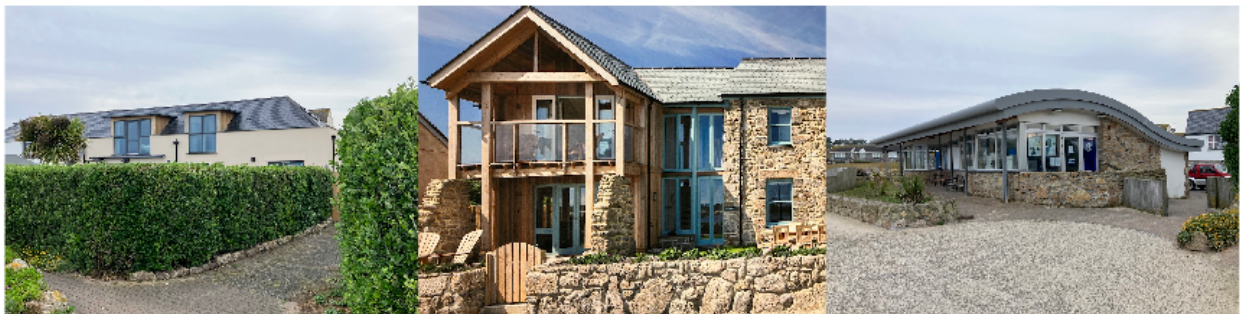
Top: 9 Little Porth. The original roof aligned with number 8 next door Below: Examples of successful contemporary designs on Scilly
