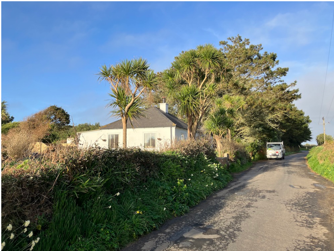
Above: View of Bishop View from the main road. The roadside boundary belongs to Bishop View. Note the establish backdrop of mature trees behind the bungalow
