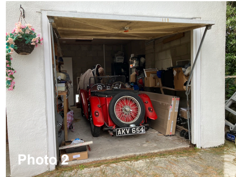
Note boarded roof slope above rafters. There is no roofing felt and, on close inspection, water marks are visible showing current leaks
