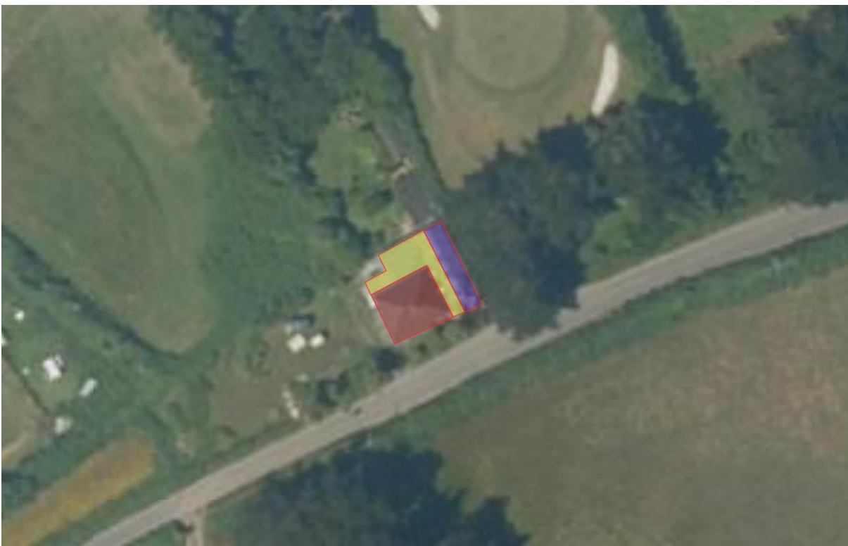
Map 02 – Showing the main hipped roof Section A (red wash) along with the pitched roof Section B (blue wash) and the connecting flat roof Section C (yellow wash). Reproduced in accordance with Google’s Fair Use Policy.
