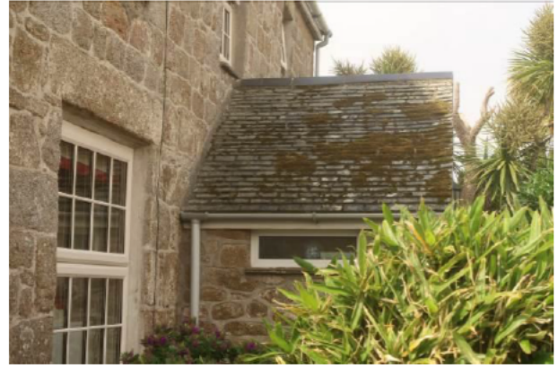
Photograph 2: Showing the porch on the northwestern aspect.
