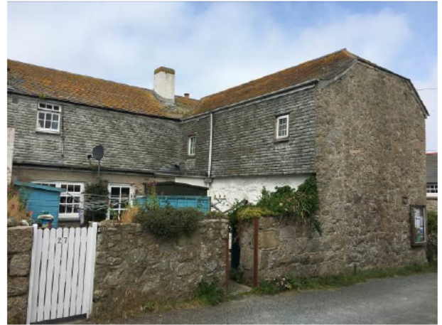
Photograph 4: Showing the courtyard on the south-eastern aspect with hanging tiles visible.
