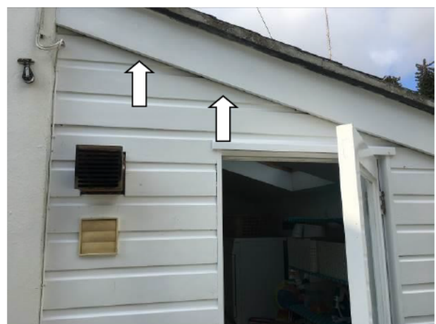
Photograph 6: Showing the access door in the lean-to component – the fascia above is indicated.
