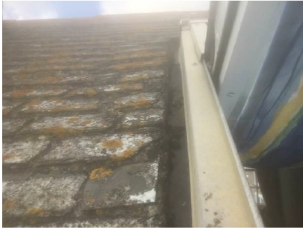
Photograph 1: Showing the tight fitting of the existing rooflight windows and adjacent wet-laid scantle tiles.
