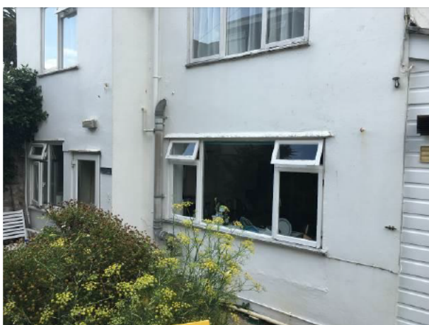
Photograph 5: Showing the southern aspect of the property – the tightly fitted uPVC windows and doors are visible.
