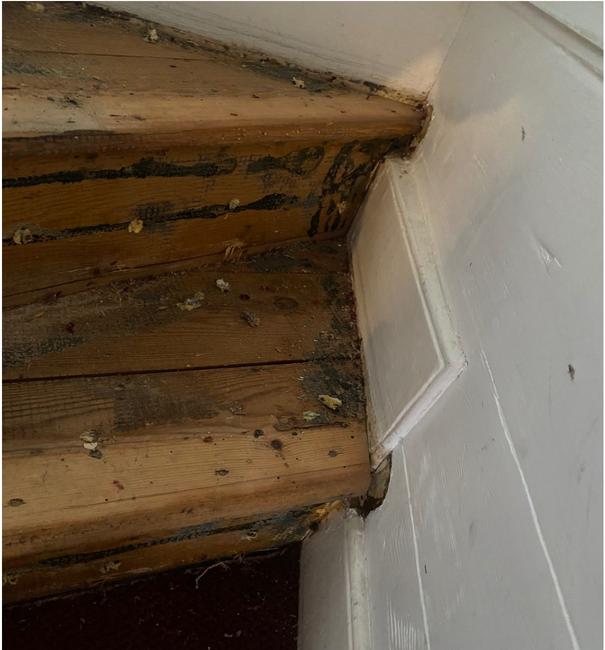
No13 Winder construction, original wall string on the left wall
