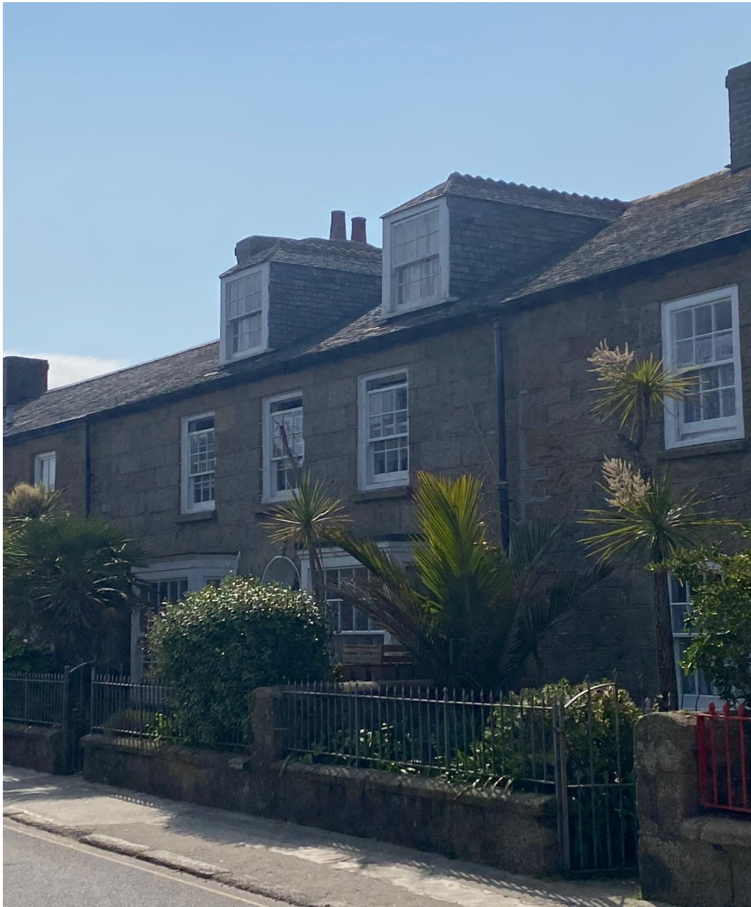
No9 Front Elevation showing the three first floor windows and the second-floor dormers.
