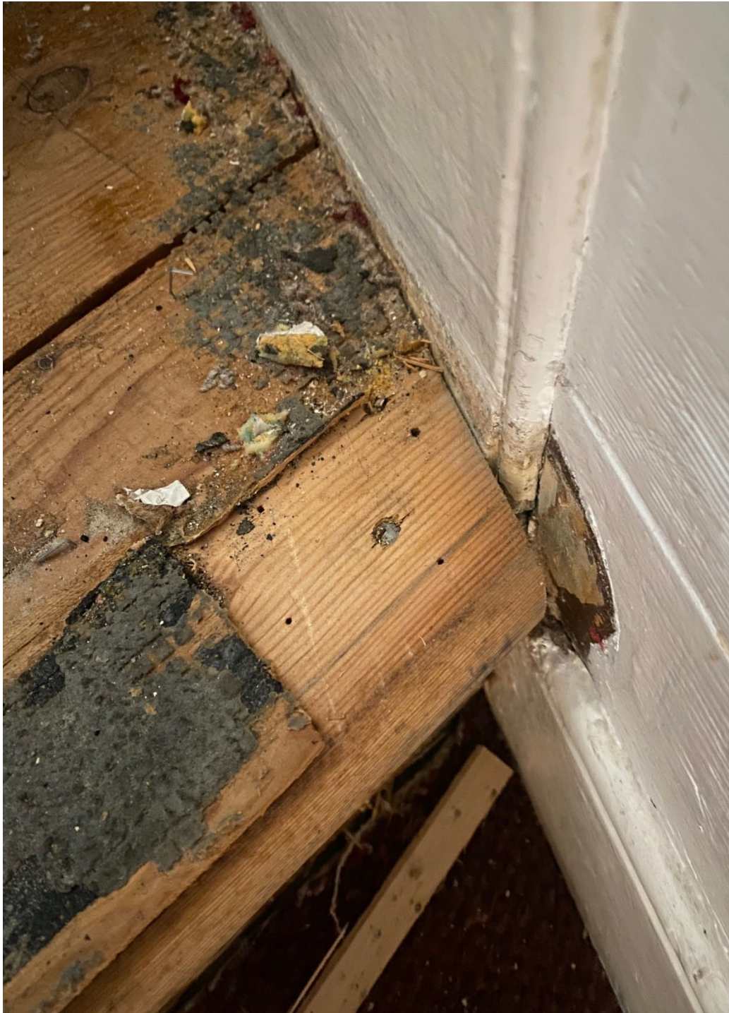
No10 Tread construction detailing the modern round head nails used
