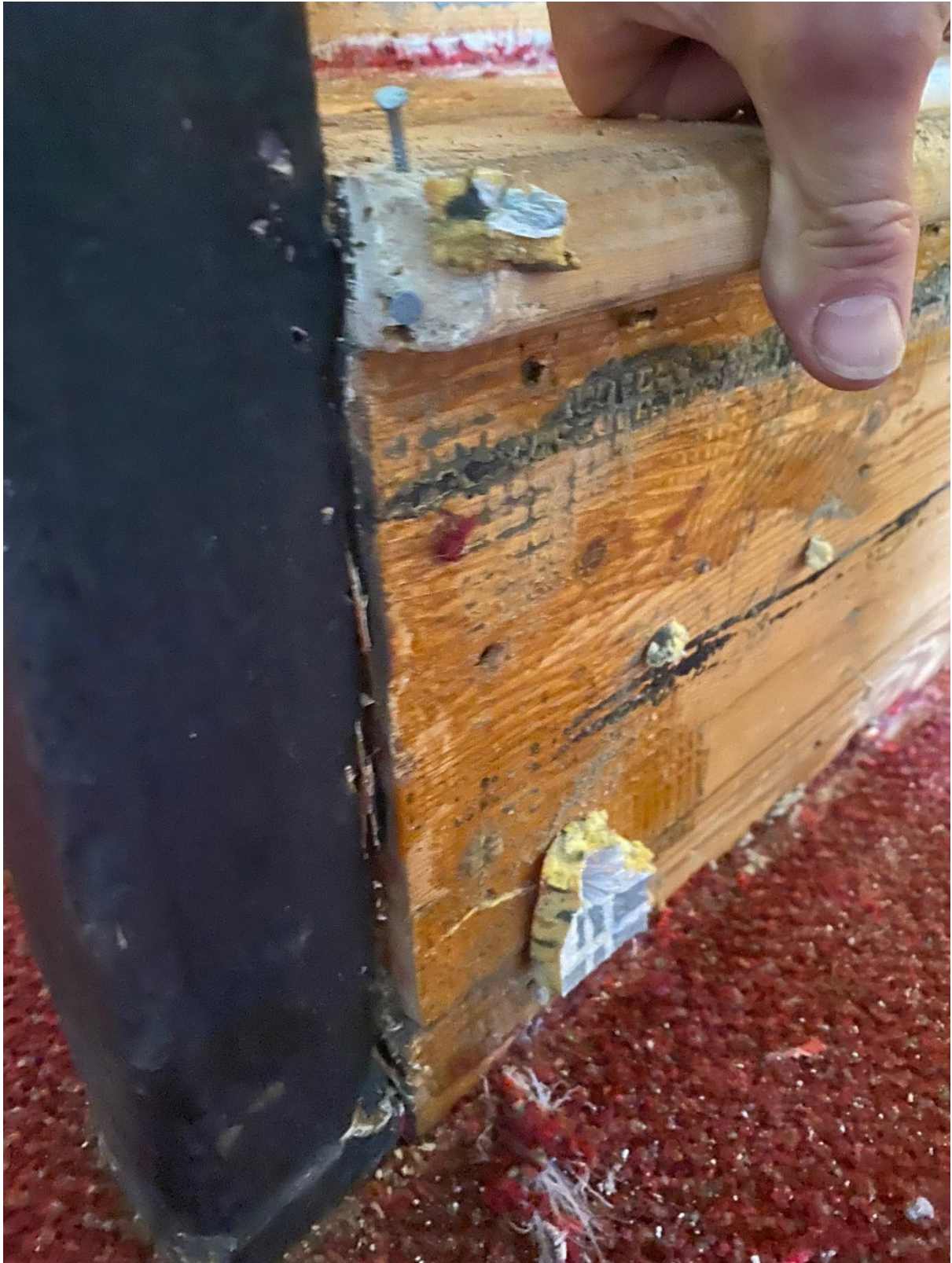
No2. This picture indicates how the bottom tread comes in front of the newel, traditionally the original riser would be housed into the centre of the newel post. The tread also extends beyond the newel.
