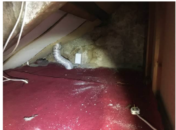
Photograph 4: Showing the typical interior of one of the eaves storage spaces.
