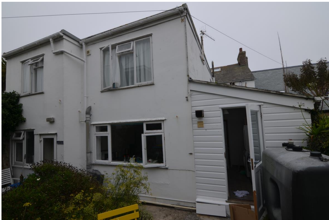
Pl.14: The southern elevations of the Rear Extensions.
