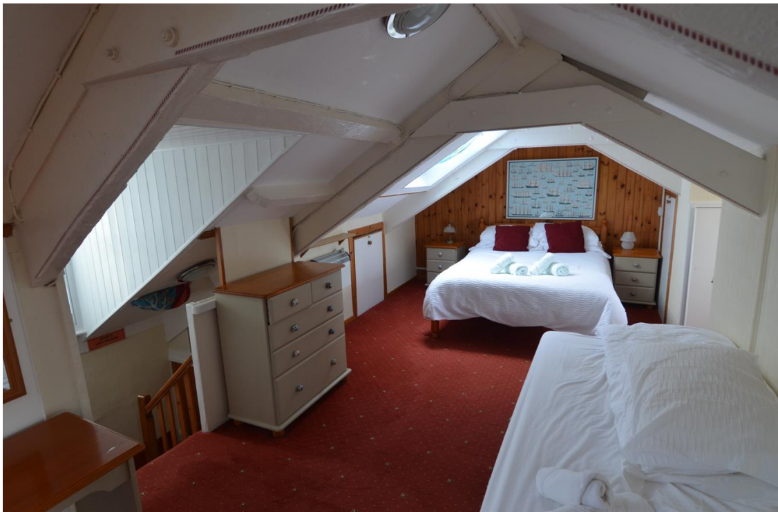
Pl.8: The attic of Wingletang, showing altered trusses.
