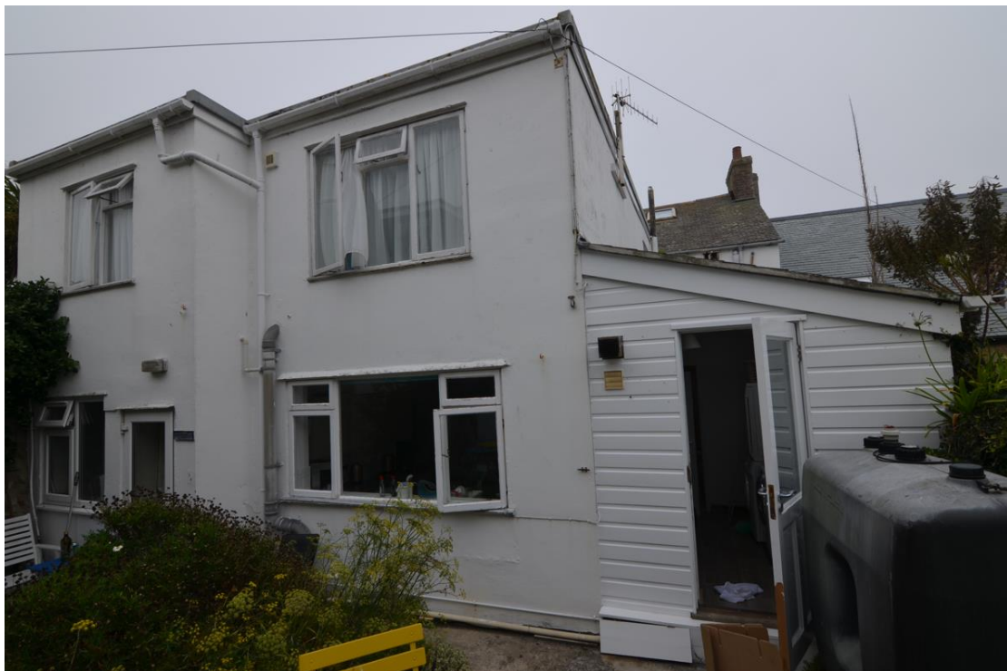
Pl.14: The southern elevations of the Rear Extensions.
