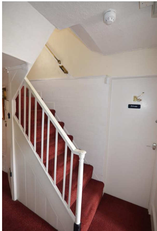
Pl.12: The base of the main stairs; note odd balusters and boxing.
