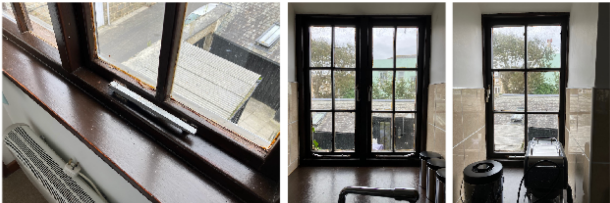
Above: Internal views of the first-floor rear windows
