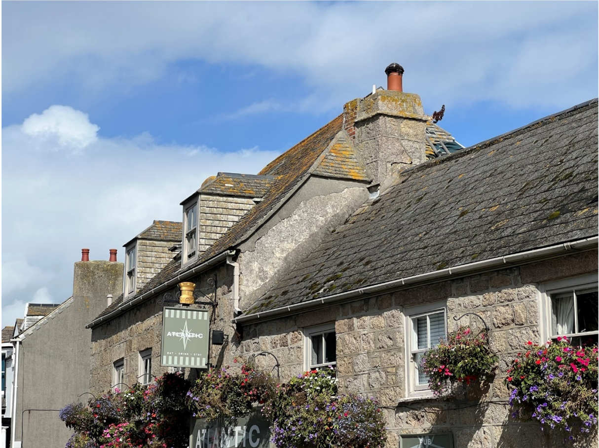
Fig 3: View of existing roof from Hugh Street.
