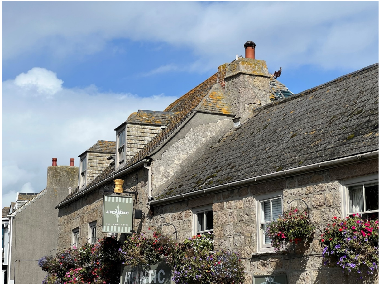
Fig 3: View of existing roof from Hugh Street.
