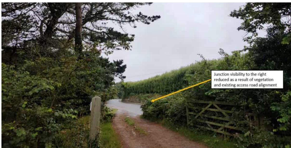
Figure 4.2: Existing site access (facing out of site to the east)
