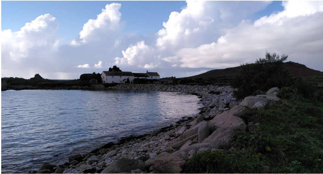
Figure 1-9: Embankment along the north of Great Porth
