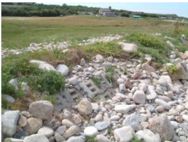
Figure 4-30: Backshore condition after winter storms (JLA 2014)
