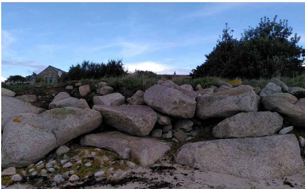
Figure 1-10: Protection provided by 1-3 tonne stones along the frontage of Great Porth
