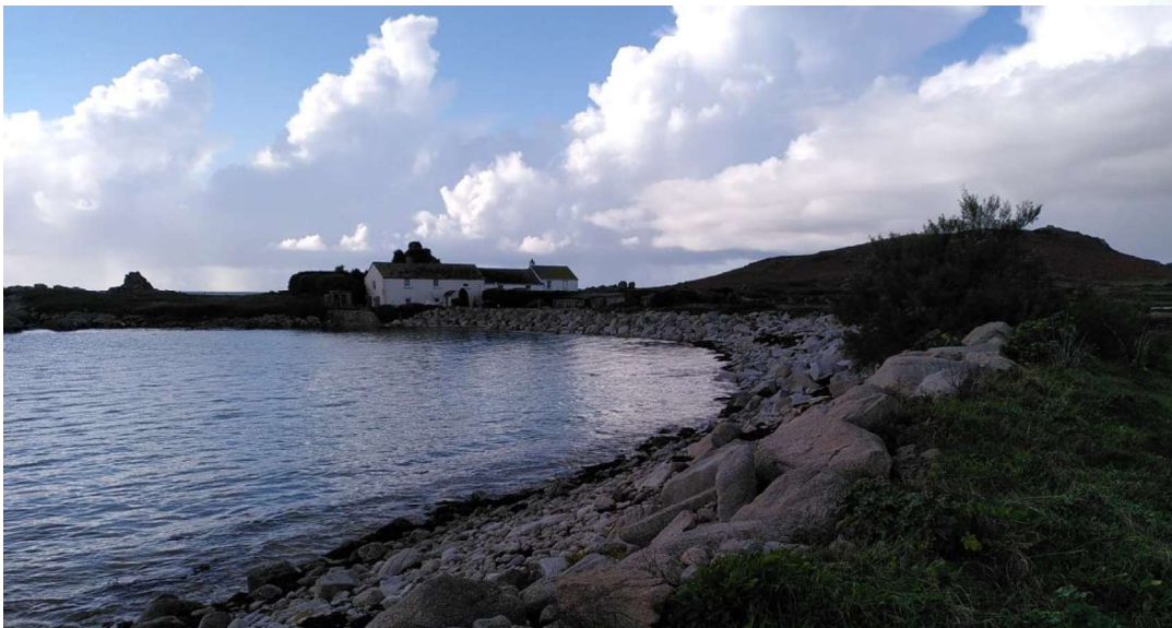
Figure 8: Embankment along the North of Great Porth.
