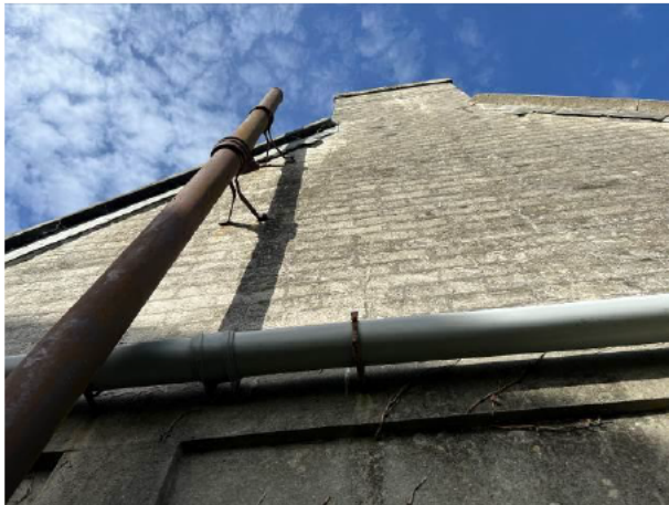
Photograph 3: Showing the southern gable of the property – there are superficial gaps behind the drop-tiles on the eastern aspect, which can be seen on the right-hand side. Those on the western aspect would not be affected.
