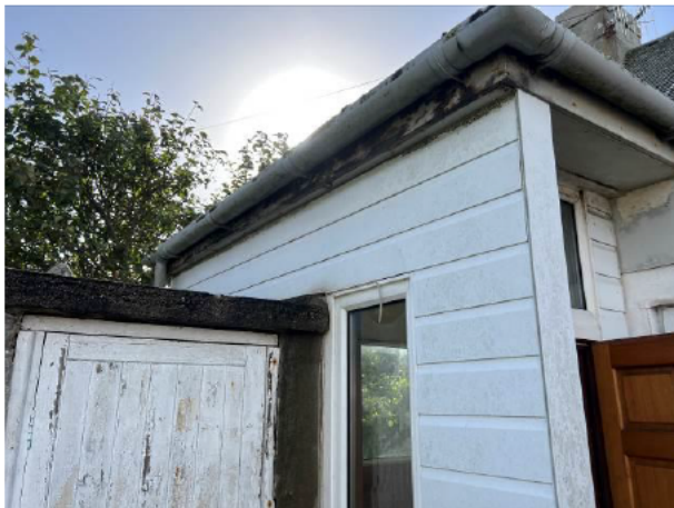
Photograph 5: Showing the flat-roof extension with uPVC cladding.
