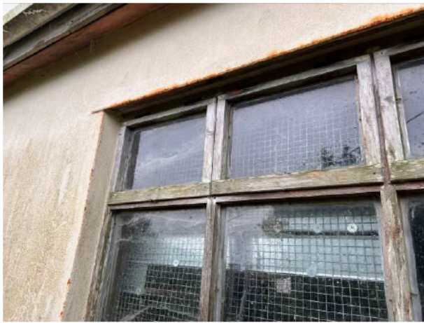
Photograph 3: Showing an example of the well-sealed window frames.
