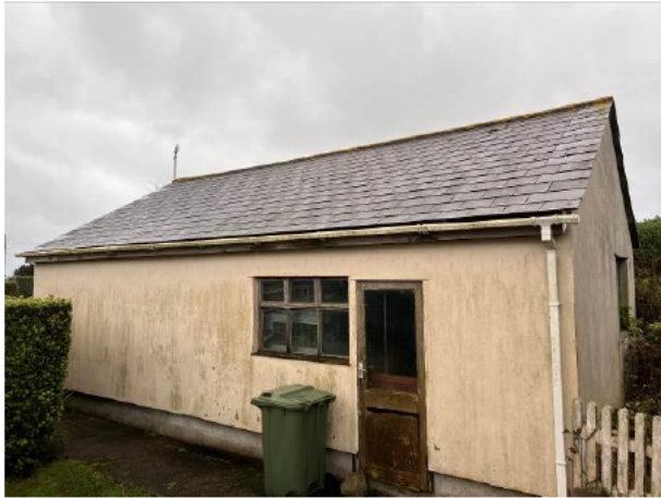
Photograph 1: Showing the northern and western (gable) aspects of the garage.
