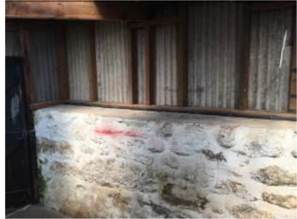
Photograph 2: Showing the typical internal structure, with the stone-block wall supporting a timber frame with corrugated sheeting attached.
