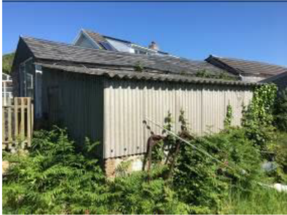
Photograph 1: Showing the northern and western aspects of the building.
