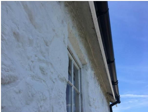
Photograph 3: Showing the well-fitted soffits supporting guttering on the southern aspect of the main building (Section A)
