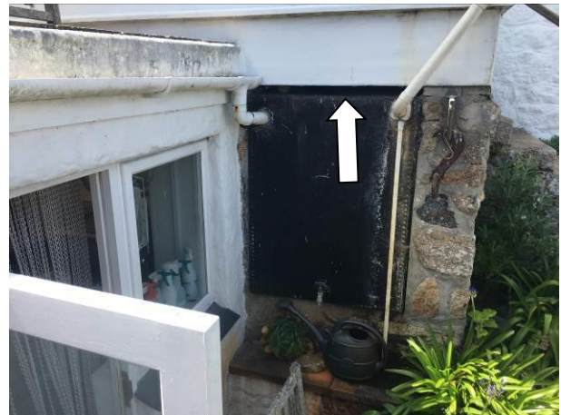
Photograph 4: Showing the integral water tank beneath the conservatory. The gap at the top providing access to the location where a historic nest was confirmed can be seen.
