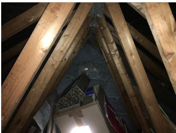
Photograph 5: Showing the interior of the loft space of the main structure (Section A)
