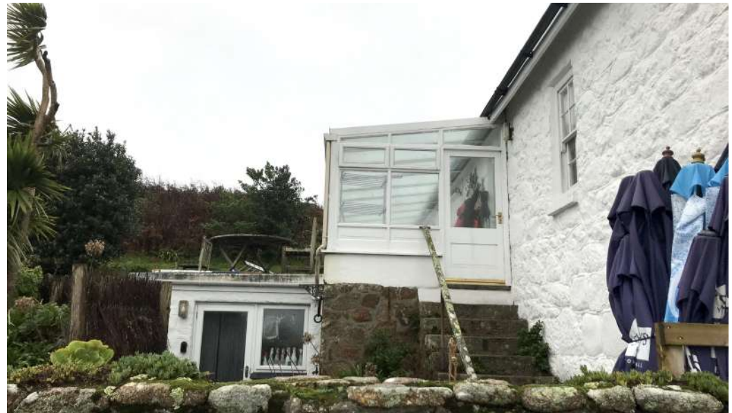
Image 9. Existing east view.
