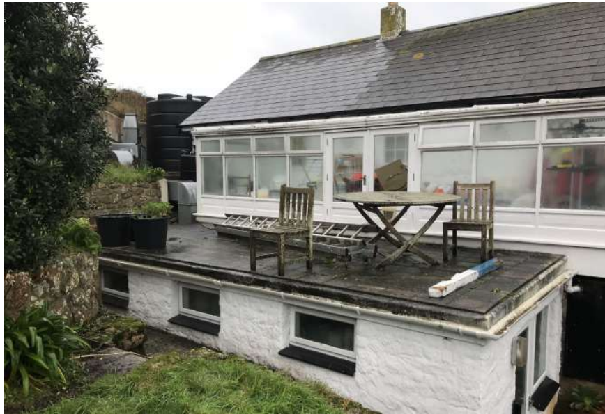
Image 6. South elevation - pub kitchen at lower level and conservatory.
