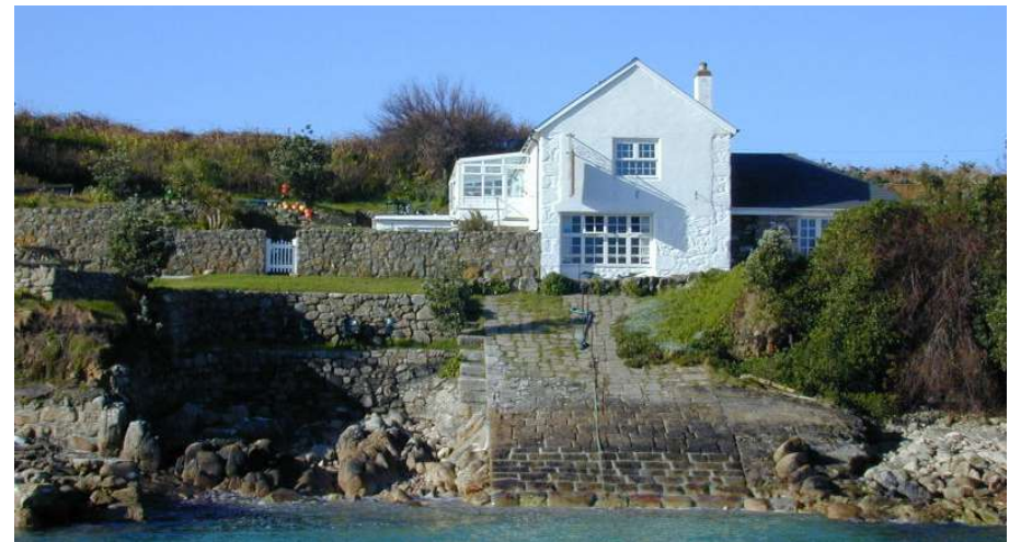
Image 2. Existing east / front view.
