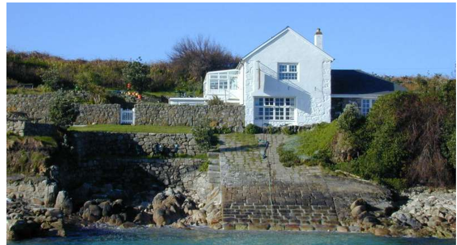
Image 2. Existing east / front view.
