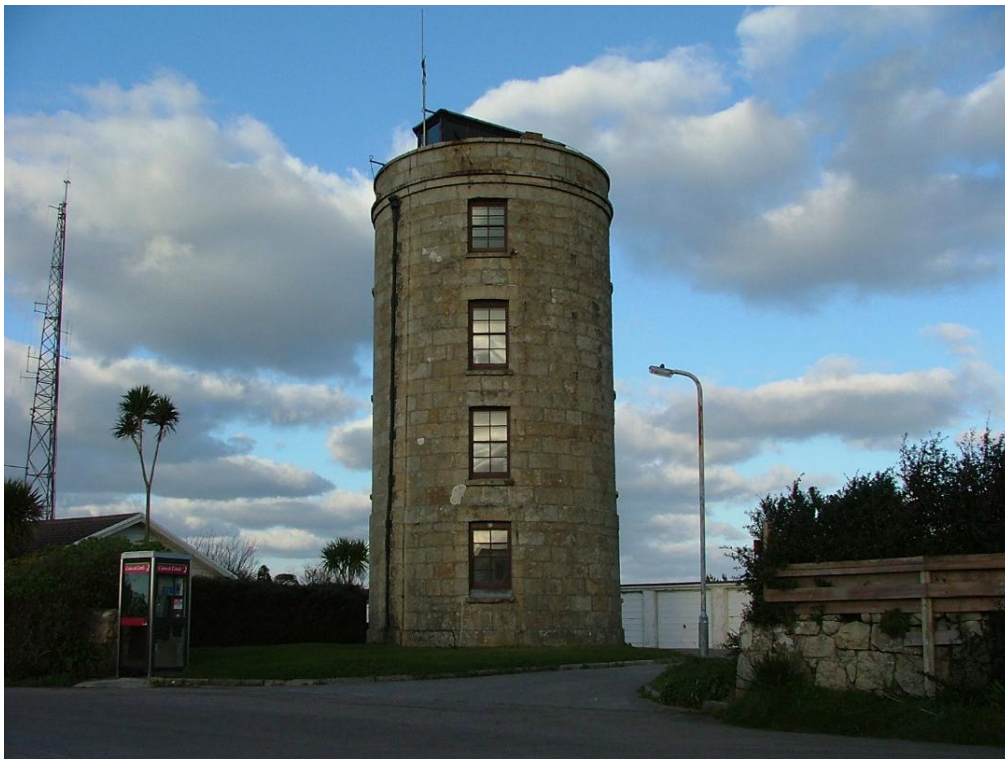
Figure 11 The Grade II Listed Coastguard Lookout Tower today, note the row of garages behind the tower (photo: Katharine Sawyer).
