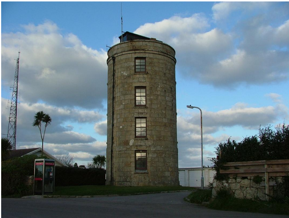
Figure 11 The Grade II Listed Coastguard Lookout Tower today, note the row of garages behind the tower (photo: Katharine Sawyer).
