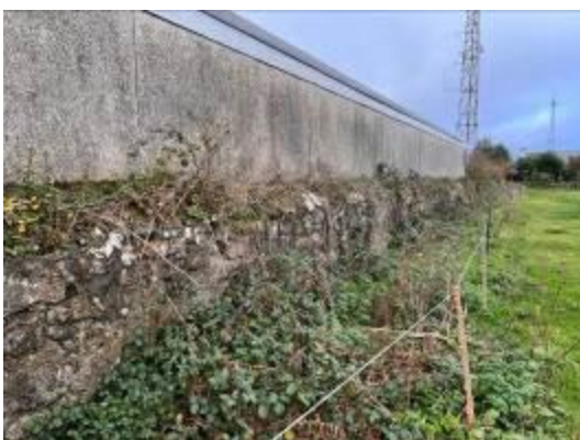
Photo 05 – Showing the western boundary wall with the offsite garage behind.
